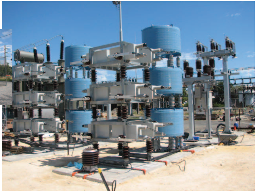
Two 22 kV 5 Mvar bank under construction
