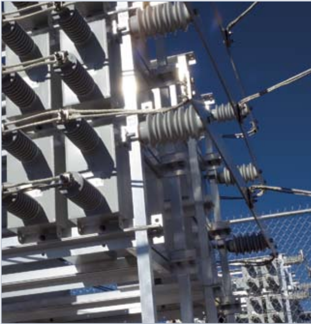
-25...+25 Mvar, 115/12,5 kV, 60 Hz, Tri-State Generation & Transmission, Clapham, USA
