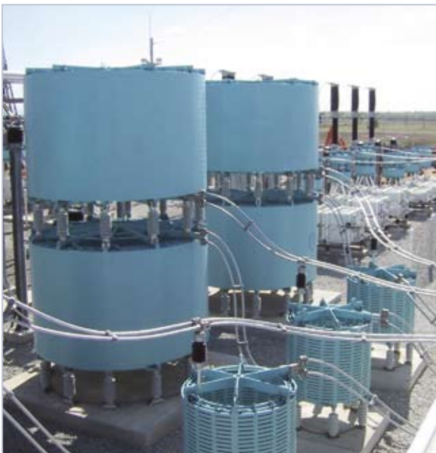
-60...+100 Mvar, 345/15 kV, 60 Hz, Campos, Furnas Centrais Elétricas SA, Brazil
