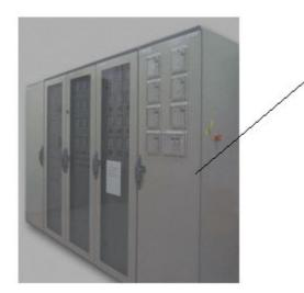
Protection and control cubicles are fastened to the floor of the building or the substation where they are located.
