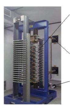
Thyristor valves (3 pieces), are brought assembled to the installation site and fastened to the floor. Their mass is approximately 1200 kg. There is one phase valve in the picture.
