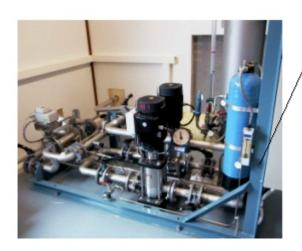
Cooling equipment is brought assembled to the installation site and it is fastened to the floor. The mass is approximately 650 kg.
