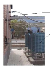
Bushing insulators are fastened to the wall of thyristor valve enclosure.
