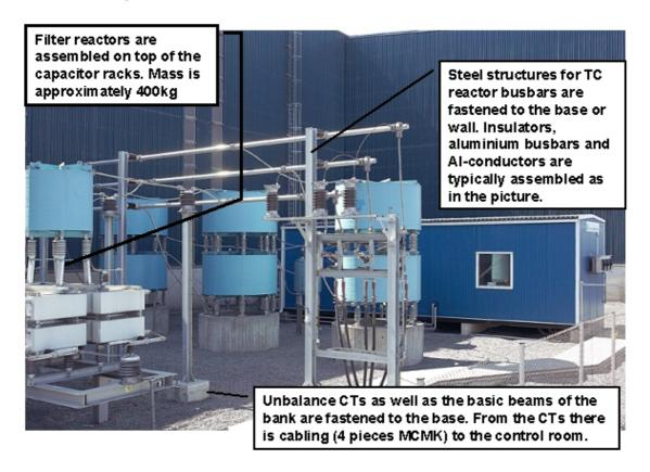
The capacitor banks have capacitor units installed in racks in our factory. Also the internal wiring inside the racks has been made in our factory. The banks have been arranged to star-star connection for unbalance protection. In series with the banks there are the CTs for short circuit and overload protection.
