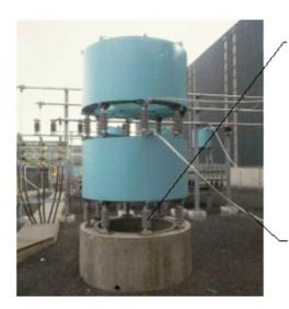
TC reactors are brought to the installation site separately and they will assembled on top of each other. One reactor weighs approximately 4000 kg. Typically there are 12 insulators between reactors.
